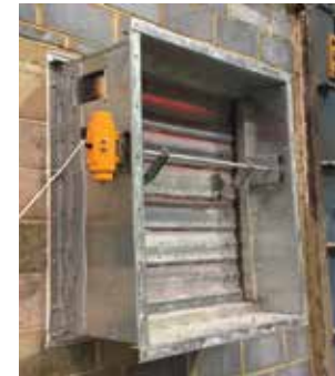
Damper Condition after 4 Hrs
