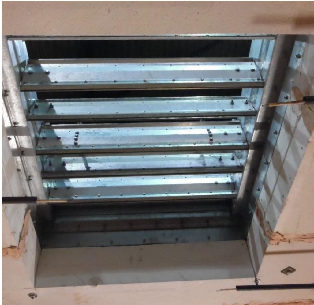
Photograph 1: Exposed face of the damper prior to test (open position).
