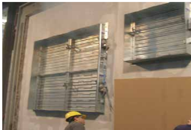
UL 555 Fire Tests - Pictures courtesy UL - USA
